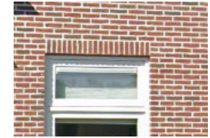
Detailering in metselwerk
